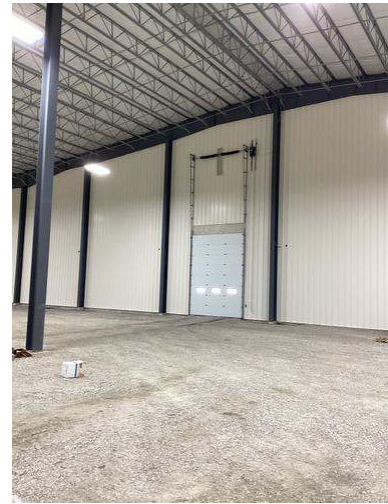
Cladding drive in door.jpeg
